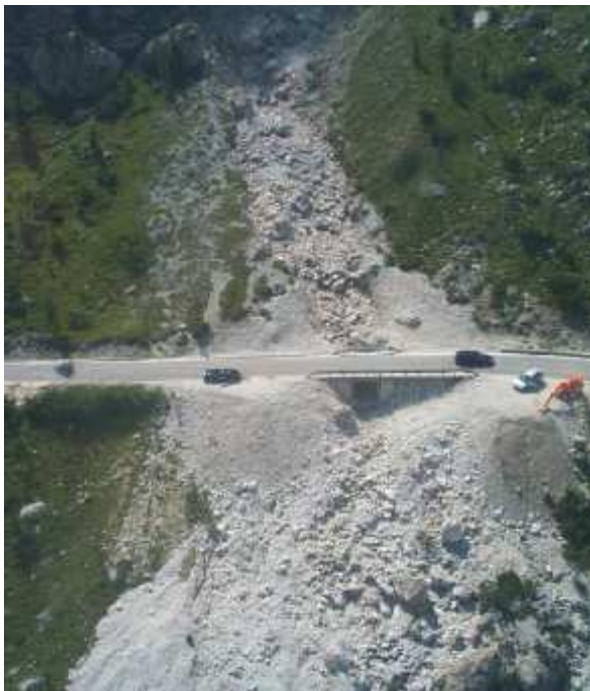
Fig. 2.25 – Deposits on the pass route to the Grödner Joch.
