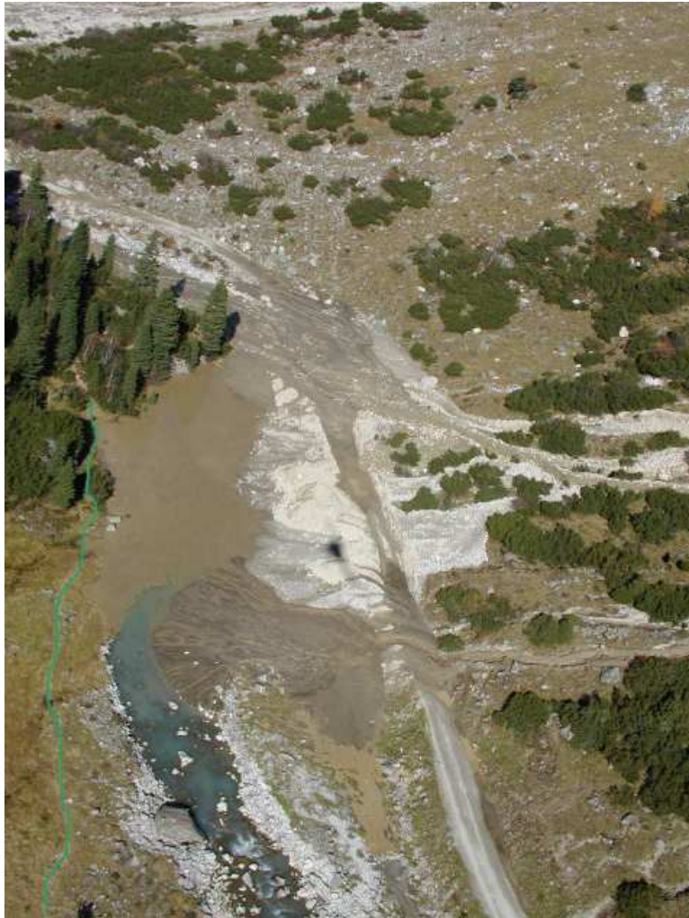
Fig. 2.32 – Debris flow over the path on the valley floor and retention of the Obersulzbach. Green line: new path.
